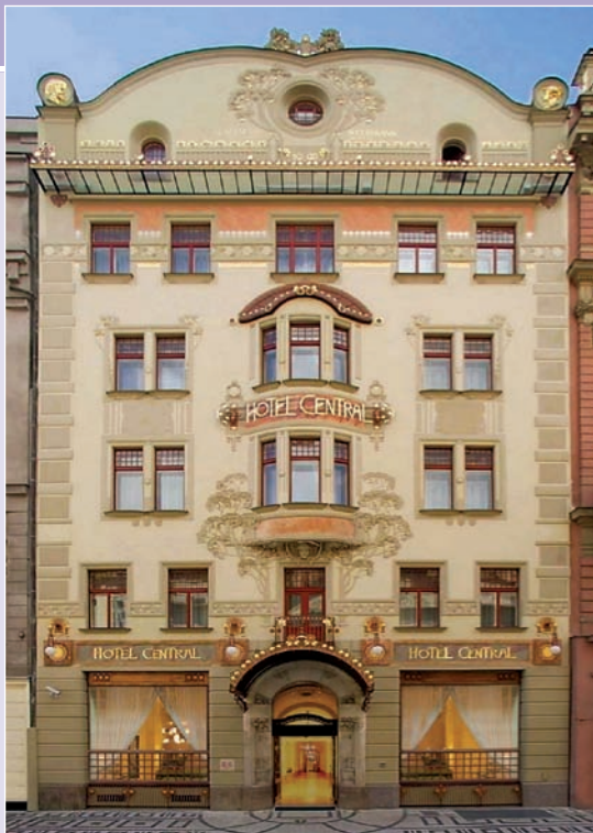
Hotel Central, classified as an historical monument, is one of the oldest Art Nouveau buildings in Prague. It is constructed with traditional materials—plaster bricks and stucco; its mauve-white hue was a popular one in fin-de-siècle Prague. The organic, tree-inspired stucco pattern, the typography chosen for the hotel's name, and the continuation of design motifs onto the sidewalk are details indicating that the building was created in a harmonious totality, in the Art Nouveau style. It is located in Staré Músto, the elegant Old Town section of the city. Photo courtesy of Hotel Central, Prague.
